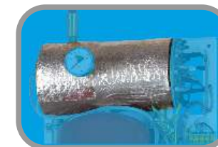
Boiler insulation mineral (Rockwool) \lambda 0,042W/mK
